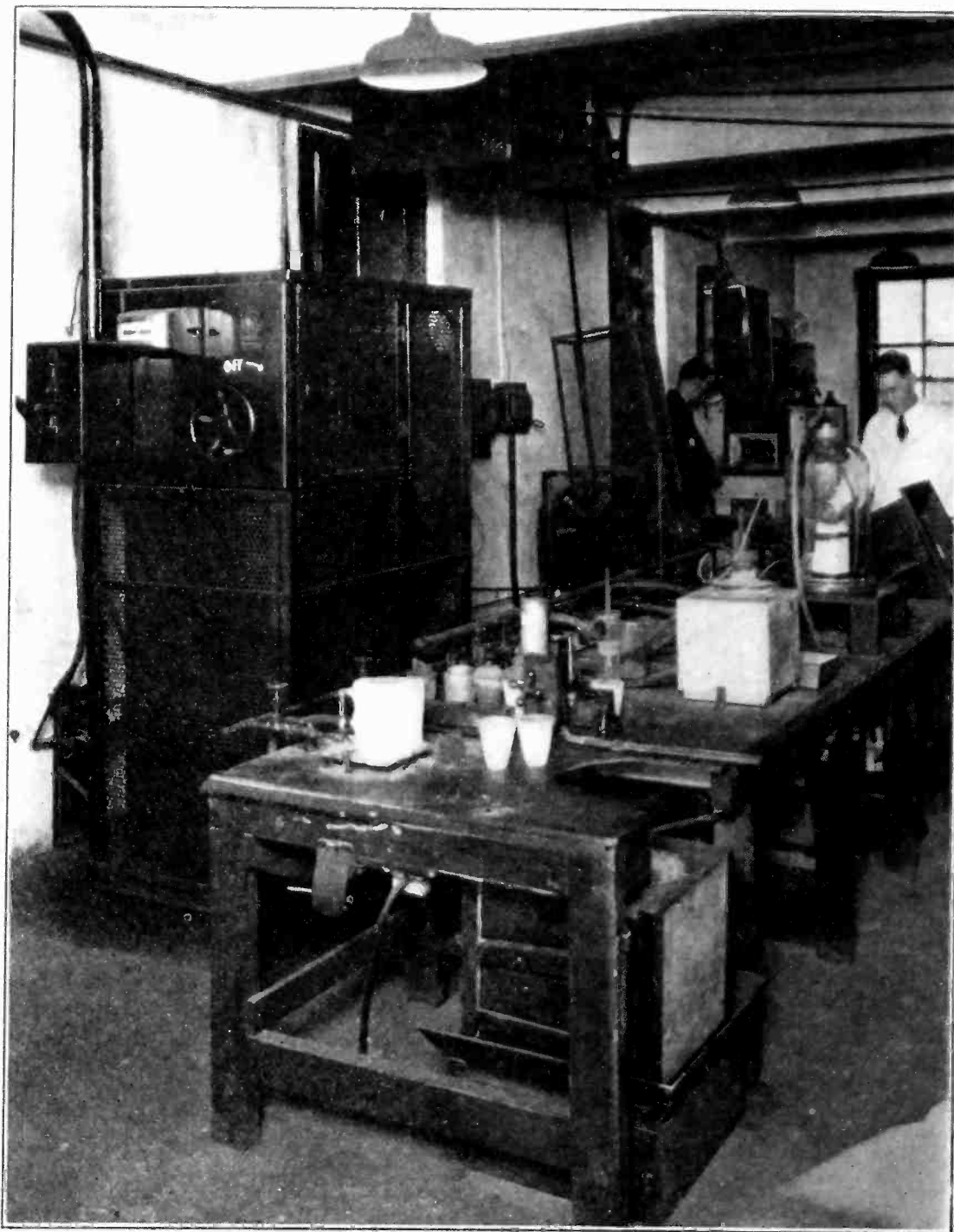
Fig. 1. Typical Installation of Small High Frequency Furnaces
