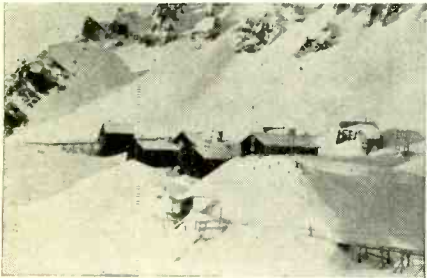
Jumbo Camp, the scene of the disaster which wiped out half the buildings of the mine, killing several men and injuring many more. The barricade, or "snow divider" at the extreme right was supposed to sidetrack avalanches but in this case the snow poured right over the barricade. K7BLI was located in the long building at the right.
