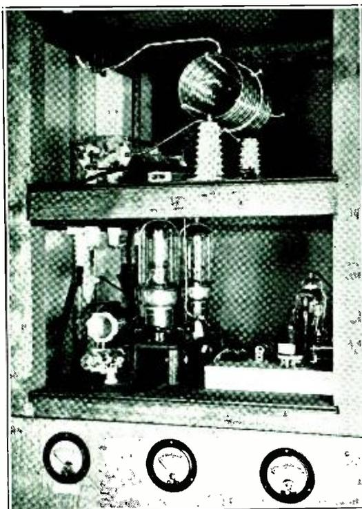
Front View of the Linear Amplifier with the Panels Removed
