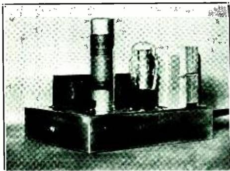
The Power Supply and Speaker Coupling Unit
