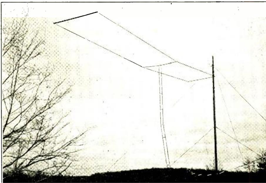
The "flat top" beam at W8JK. Used on 14 Mc., it is less than 60 feet long.
