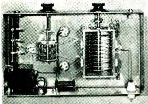
Bottom view of amplifier showing grid and plate tuning condensers.
