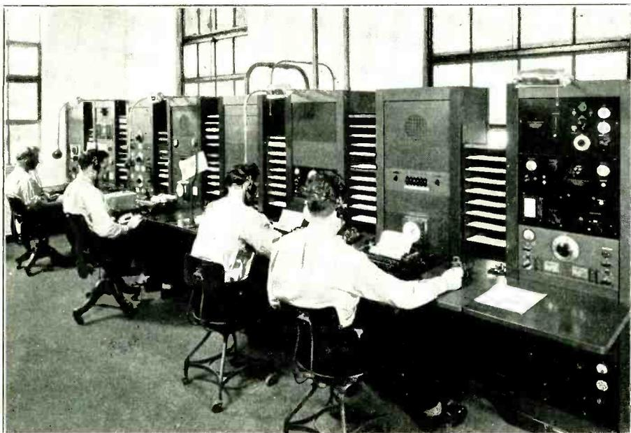
E.A.L. ground station at Miami, Fla. Transmitters are remotely controlled. The unit to the extreme right in photograph is the frequency standard used for periodic checks upon the equipment.
