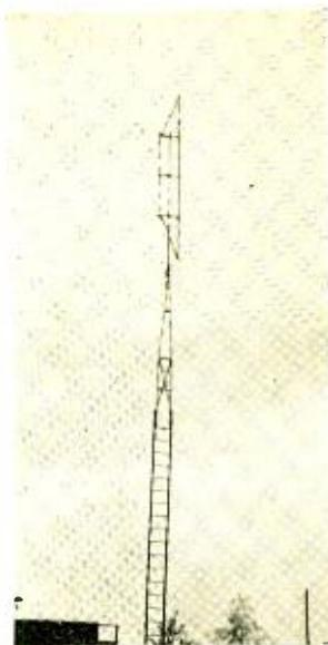
The co-phased, co-linear vertical array in use at W8VO, Akron, Ohio. W8VO was successful in contacting W6PEX in Alameda, California, for his eighth district on 56 Mc.
