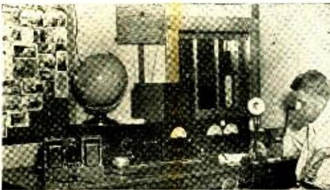
The operating position at W9ARN showing the OM to the right and the unfinished direction indicator for the rotatable beam at the top of the picture. The crank for turning the beam can be seen just below the mike.
