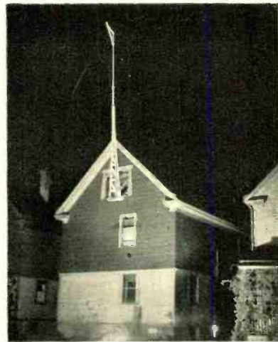
The mast at W8IPD is easily lowered. A block and tackle system into the attic makes it possible to lower the mast and make antenna adjustments with little loss of time.
