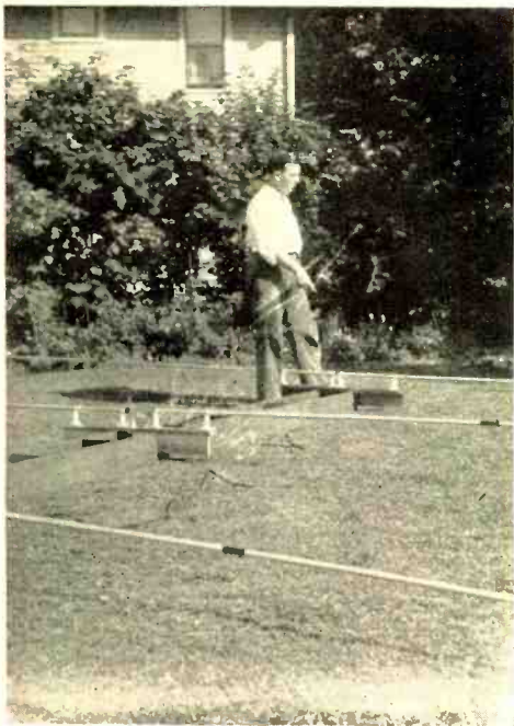
Figure 3. The three-element beam being assembled on the ground, as pointed out by Dr. Dodds, W9ELK.
