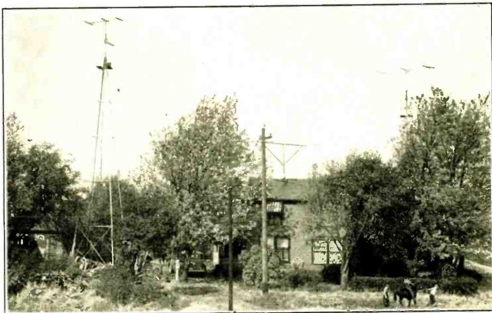
W9ZHB, Zearing, Illinois. The beam of the left is for 56 Mc., the one mounted upon the house in the center is for 14 Mc., and the one above the trees on the right is for 28 Mc.
