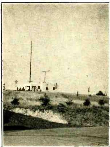
The location of W8CIR. A 3/2-wave vertical is located atop the telephone pole and a 7-element Yagi mounts on the rotary affair on the roof.
