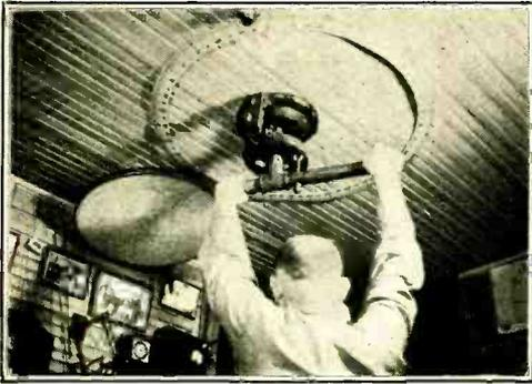
Ed. Grabill rotating the antennas at W9ZHB. All three antennas are turned simultaneously by moving the lever.
