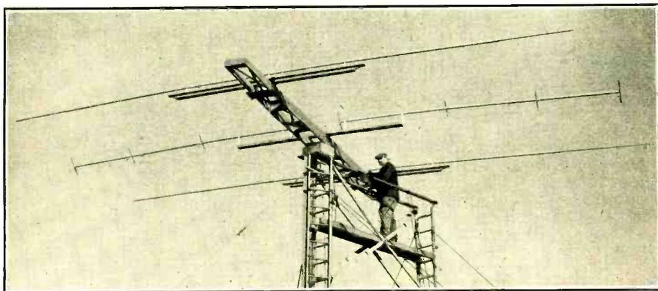
Figure 1. 3-band rotary antenna at W8JK using 4-wire doublet as driven element.
