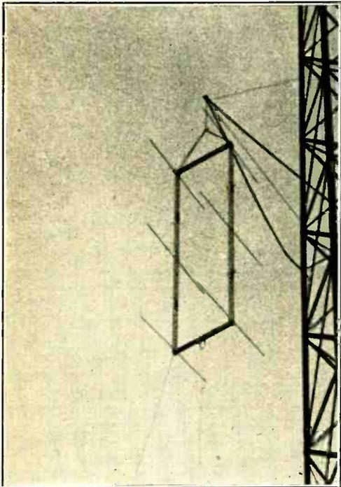
The stacked array at W9CLH. This antenna is supported 100 feet in the air from the side of a b.c. station tower.
