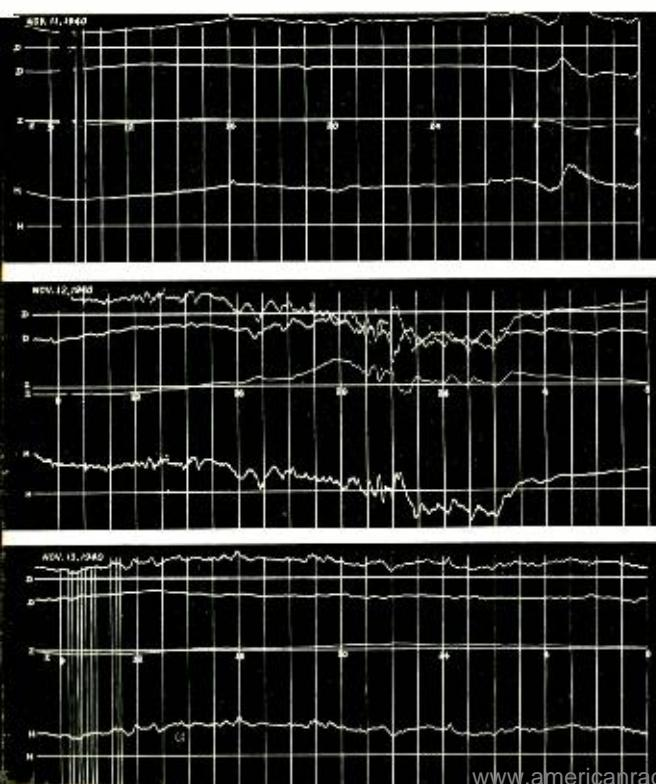
Photostats of curves traced by the new Eschenhagen Magnetograph at the Cheltenham, Md., observatory of the U. S. Coast and Geodetic Survey for the period of November 12 to November 14, 1940.
