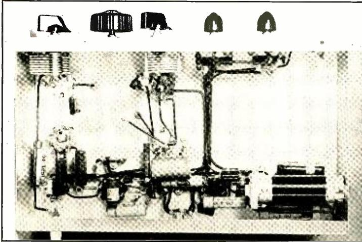
The under-chassis view of the super shows the straight-forward placement of parts, and the neat wiring installation.
