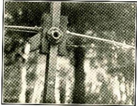
Detail of center portion of boom, showing reinforcement, method of attaching bamboo elements, and floor flange for fastening to pipe support. With heavier bamboo, the truss wires would not be required.
