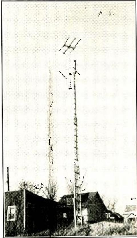
The 56-Mc. horizontal and vertical 56-Mc. antennas in use at W9QCY.
