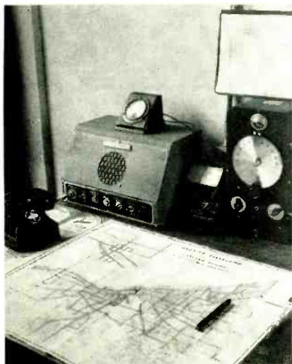
The G-E 25-watt 2-way f-m communication equipment on desk of dispatcher of the Cleveland Railway Co.
