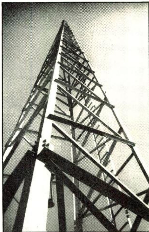
One of the 120-foot vertical towers forming a part of the radio range station.
