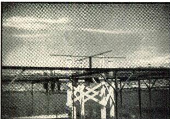
Close-up of the radiating system of the 75-megacycle "Z" marker station, with its four horizontal dipoles. See Fig. 2 for pattern.
