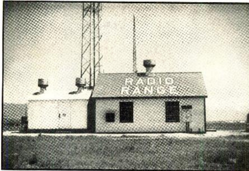
CLOSE-UP OF THE FIVE-TOWER RADIO RANGE STATION.
