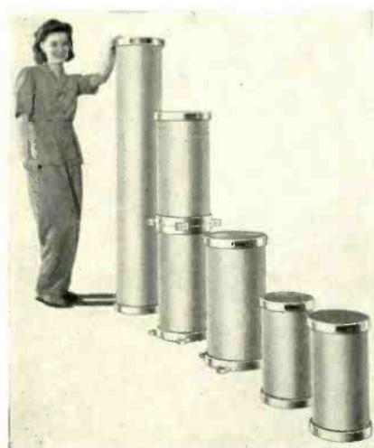
strength and maximum safety from external flashover. Long creepage path between terminals means an exceptionally conservative and safe rating for these units. Dependable operation and long service life is assured at rated voltages and ambient temperatures up to 65° C.
