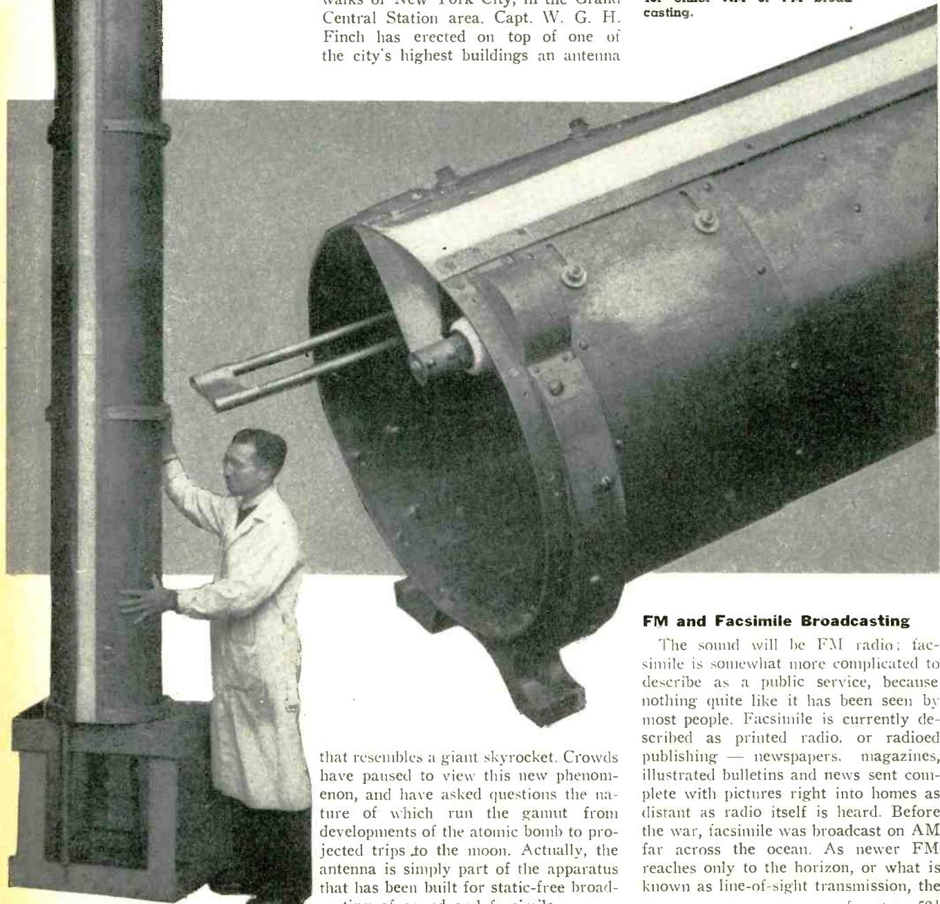
that resembles a giant skyrocket. Crowds have paused to view this new phenomenon, and have asked questions the nature of which run the gamut from developments of the atomic bomb to projected trips to the moon. Actually, the antenna is simply part of the apparatus that has been built for static-free broadcasting of sound and facsimile.
