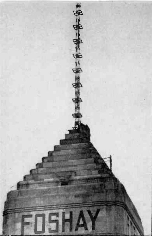
The world's first permanent super-efficient FM antenna erected by Radio Station WTCN-FM atop the Foshay Tower, Minneapolis, Minn. The eight-element square-loop antenna and FM broadcast transmitter installed by WTCN-FM were manufactured by Federal Telephone and Radio Corporation, associate of the International Telephone and Telegraph Corporation. Radiated power is 400 kw.
