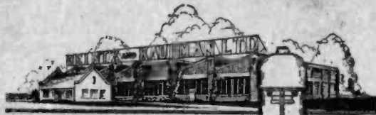
MAIN PLANT BUILDINGS
