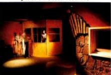
suring about 400 square feet (37 square meters) and has a seating capacity of 15. There is carpeting, wall-to-wall. The back wall is a convex, horizontal broad-band wood slat resonator. The power switches are cleverly concealed behind the wood slats. All surfaces are durable and are done with local materials, except the wood, which is clear fir imported from Norway. All the woodwork and detailing is precise and clean.
