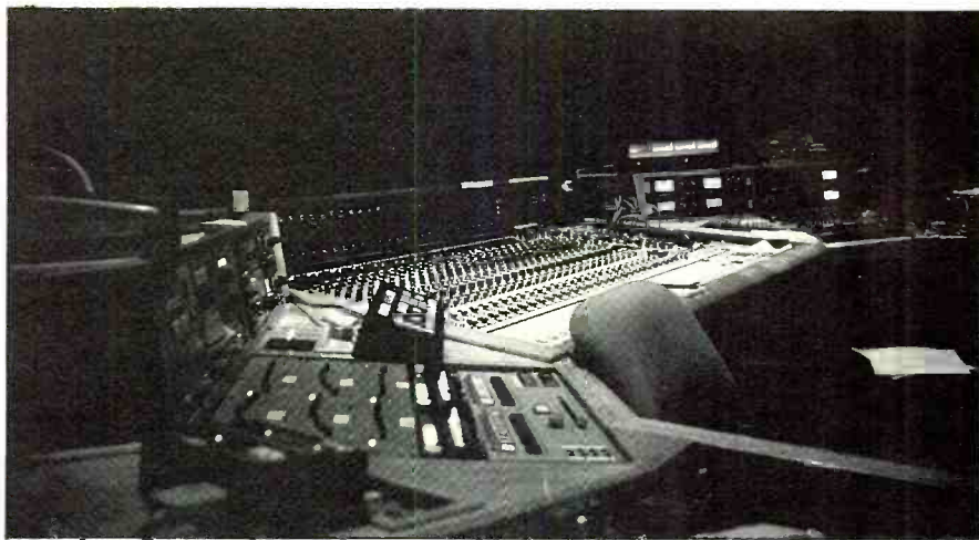
Zoetrope Studios’ re-recording stage built for the mix of “Apocalypes Now”. Acoustic design © by Jeff Cooper.
