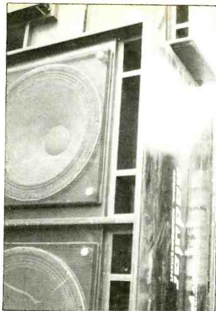
Figure 4: The "Multiple Warhead" enclosure, loaded with JBL K151 18-inch drivers, is constructed of a wood-chemical hybrid material that reportedly offers a high rigidity factor.
