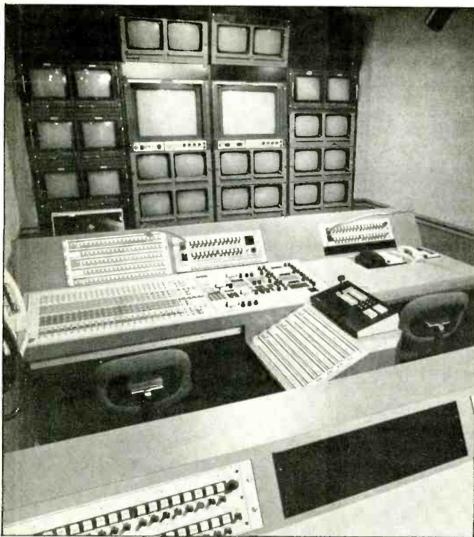
The Video Production Area (left) house a Grass Valley 300-A-3 Series video switcher, and an Ampex ADO Digital Video Effects Unit; the Videotape/Chyron Graphics Generation Area (right) serves as home for Ampex VPR-2B one-inch, C-Type videotape machines, with full timecode and Slo-Mo capabilities.
