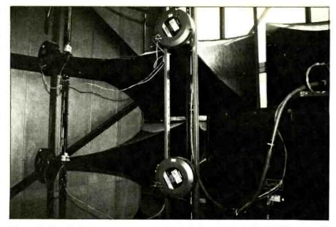
Figure 3: The Coliseum system comprised 16 Panasonic WU-S948P horns, 12 WU-S968P twin-Bessel horns, and 24 RAMSA WU-S907/8WP 15-inch waterproofed loudspeakers.
