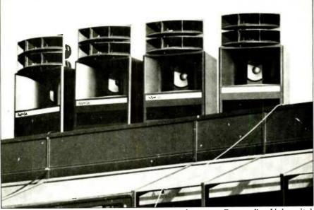
Figure 10: Roof-mounted RAMSA loudspeaker clusters at Pepperdine University's Raleigh Runnels Memorial Pool, where 5,000 spectators attended Olympics water polo events. The sound system was operated by the event commentators.
