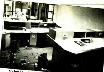
Video Production Control area prior to the fitting of various video switchers, monitor and routing controllers.
