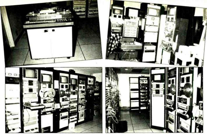
A central video prelay, layback and film-to-tape transfer center currently houses the facility's Sony PCM-3324 digital multitrack (top-left), plus Sony JH-110 eight-track and one-inch C-Format VTRs (top-right). A larger rack bay (bottom-left) houses additional VTRs and VCRs, plus video switching and distribution hardware. A companion video machine room on the facility's second floor (lower-right) links various production areas via audio, video and machine-control tie lines.
