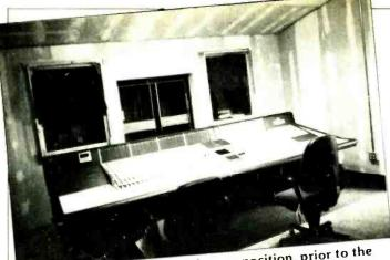
The SSL console in its final room position, prior to the installation of monitor loudspeakers and central racks.
