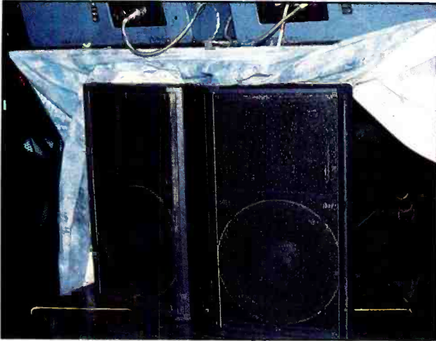
Figure 8. DeltaMax cabinets were used for near-field coverage of the forward seating areas.
