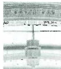
Carnegie Hall A coherent array of UPA-1A loudspeakers, supplemented by MSL-3s and 650-R2 subwoofers (not pictured), is permanently installed for live performance reinforcement.
