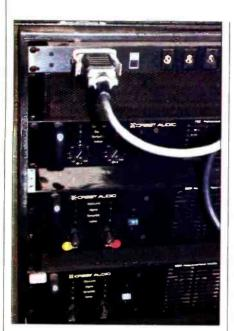
Figure 1. A custom "steering box" allowed the amp racks to be switched to the left or right mains without repatching.
