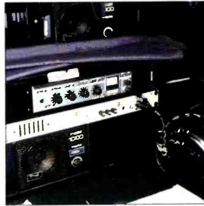
Figure 3. The conductor's position is equipped with a private mini-monitor system using Anchor-powered speakers and an intercom control station.
