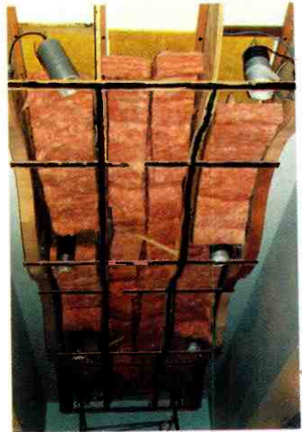
Skeletal view of studio diffusor cloud showing ribs and damping material.
