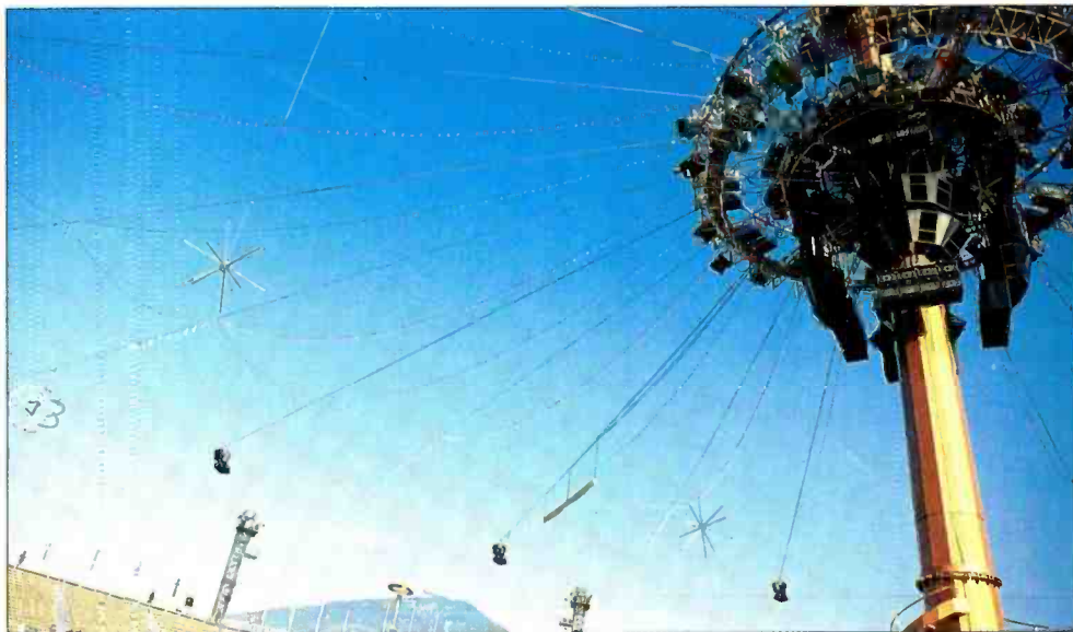
The central production mast showing U.S. Sound's loudspeaker arrays for 360° coverage. Additional signal-delayed speaker units were suspended from support cables anchored to the stadium perimeter.
