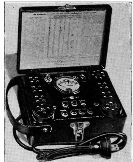
When it comes to tube checking, both instruments are the same, so we shall confine ourselves to a description of the H-33. This unit, it will be seen, has eight sockets mounted on the sides of the panel. These will accommodate all type tubes, including the new 6- and 7-prong tubes. The 7-prong socket will handle tubes with a filament or heater voltage of either 2.5, 6.3, so that any new tubes which may be an-
