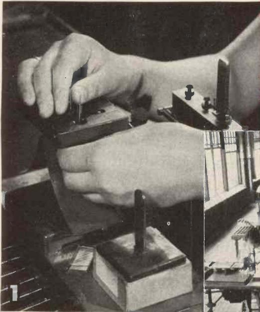
(1) Gauging grids. This operation is typical of the scores of painstaking measurements and tests conducted in the Paris Assembly Section. (2) A view of the General Assembly Section. Here the mounds are assembled before being
