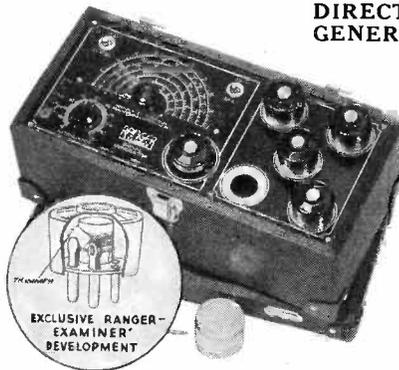
Model 557 has the same features as described for Signal Generator Model 540 except that it is installed in a black leatherette carrying case and is an integral part of the case. The five individually calibrated coils are nested on the side as shown, handy for instant use. The attractive panel is silver and black.
