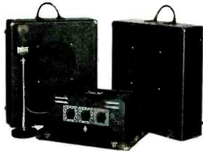
the two electro-dynamic speakers which are included with it. It can also be used with permanent magnet dynamics.
