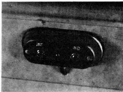
Fig. 4. Exposed type outlet unit mounted on window sill.
