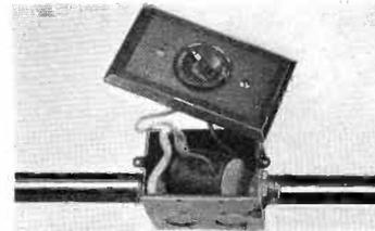
Simple exposed wiring for existing apartment houses; concealed BX or conduit for new apartment houses; or knob-and-tube for private residences.
