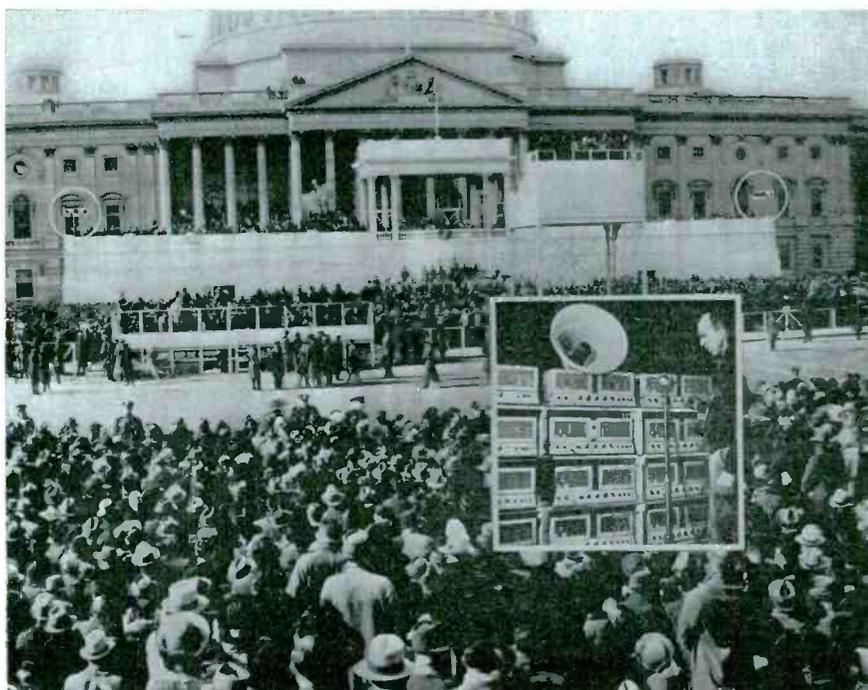
perienced. The trumpets were mounted in pairs on poles erected on each of two corners of the speaker's stand, fanned out to cover the rear of the crowd, to avoid excessive volume for those in
