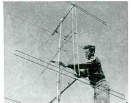
Vertical mast and cross-arms of antenna of Perma-tube (electricweld steel tubing coated with a plastic type rust-resisting finish) developed by Jones & Laughlin Steel Corp.
