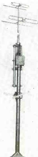
Crown antenna rotator mounted on a Camburn jack-up TV tower. The jack-up tower is said to have a variable height of 20' 8" to 47'.
