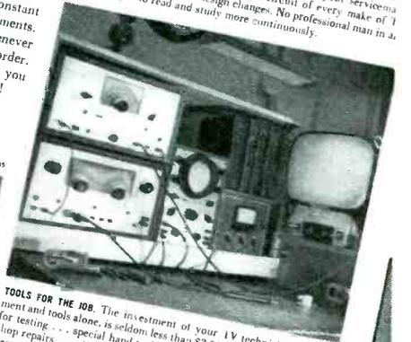
**TOOLS FOR THE JOB.** The investment of your TV technician in equipment and tools alone, is seldom less than \$3,000. Precision instruments for testing . . . special hand-tools . . . bench equipment for major TV shop repairs . . . these are pluses he must add to the customary house-nessman's investment in shop and trucking facilities.
