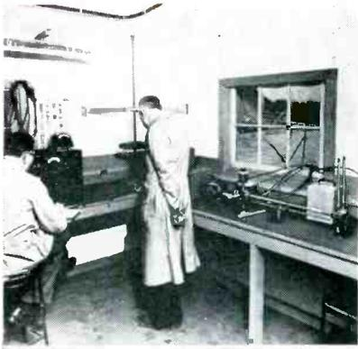
Antenna research laboratory recently set up by Ward Products Corp., in Ashtabula, Ohio, for the design and testing of TV and automotive antennas. According to W. H. Rickards, Ward director of engineering, test facilities include equipment for the measurement of impedance,  $V_{SWR}$  and gain. A pattern range has also been constructed in the lab.
