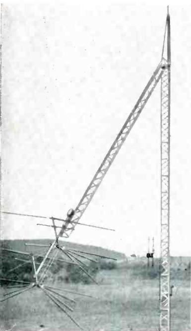
**4.** Attach an **ALPRODCO ROTATOR** if available, and an **ALPRODCO ANTENNA**, and it's all ready to go up. Pull the antenna away from the tower base to get winch leverage and crank.
