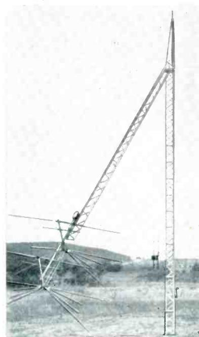
**7. REPAIRS?** If you haven't used an Alprodco Antenna and rotator, most likely there are repairs to be made soon. So—in 10 seconds you can lower the antenna to a handy working position. All done? Up she goes!
