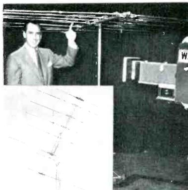
All-aluminum single-boom vhf fringe antenna, using 24 elements on high band and seven elements on low bands, introduced recently on a national TV program. All elements are in same plane; said to require no boom braces on 1 1/4" crossarm. Assembled by means of spring-loaded quick-rig design. Incorporates penta-phase principle, said to overcome loss of signal because of wave distortion. (Super Trapper; Technical Appliance Corp., Sherburne, N. Y.)
