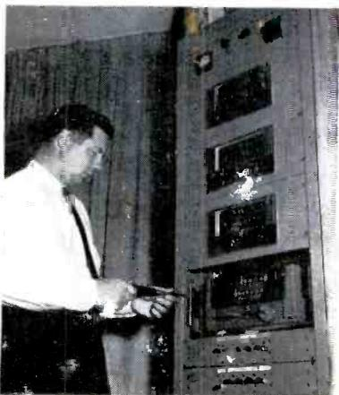
**INSTALLING TUNER-AMPLIFIER** in sound-system cabinet used in Trenholm system.
