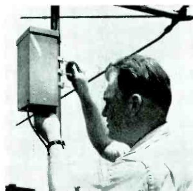
**INSTALLING** a mast-mounted preamplifier.
