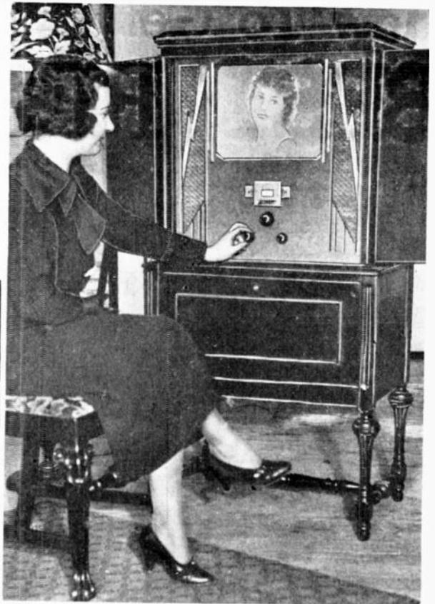
Photo above shows the new Farnsworth Television receiver developed in his Philadelphia laboratories and it is very interesting to note that the girl's face reproduced on the screen is the actual reproduction from the Farnsworth special cathode tube, and not merely picture painted on it by an artist. Photo at left shows Farnsworth Television pick-up at studio.
