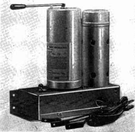
Commercially available beat oscillator which can be used in conjunction with any super-het as explained in this article.
