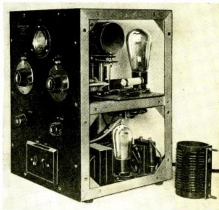
The photos above and at left illustrate the simple, business-like appearance of the 10-watt universal short-wave transmitter. It is provided with simple switches for changing from C.W. (code) to phone transmission. Ordinary tubes such as those employed in receivers are used, viz.: two 1Z pentodes, one '24 screen grid tube and an '80 rectifier.
