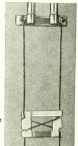
Dimensions of a lead-in constructed on the new type "Q" system is shown at left. Above—Transposition block in position.
