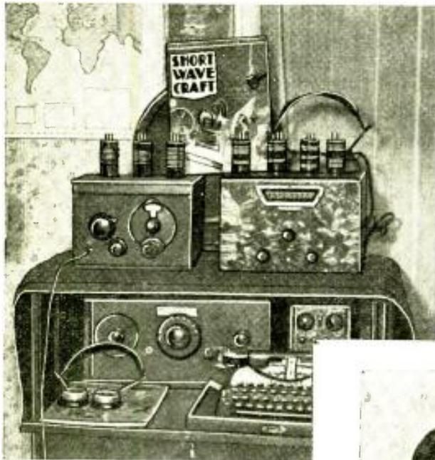
GLOBETROTTER: this works fine. The set on the right is a three-tube ALLEN. This works better than any of the others that I have built as yet. The one inside the cabinet is my "old faithful"—it has three tubes—35 Det., 27 and 45 output. The power supply on the right supplies the set in the cabinet.
