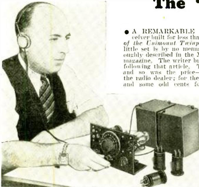
● A REMARKABLE "2-tube" short-wave receiver built for less than \$5.00. That is the story of the *Unimount Twinplex*. The circuit of this little set is by no means new, having been thoroughly described in the March, 1934, issue of this magazine. The writer built the "B" Twinplex by following that article. The results were splendid and so was the price—from the viewpoint of the radio dealer; for the author had spent \$15.00 and some odd cents for the component parts.
