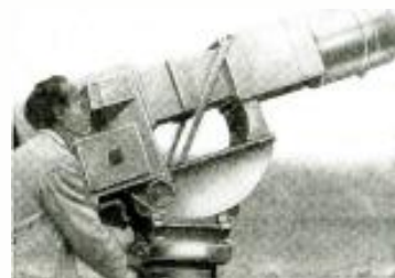
← Left—The television camera equipment with huge telephoto lens used to focus objects clearly even 400 feet away.
