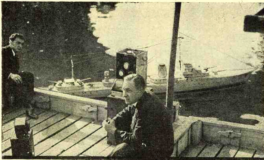
This photo shows model warship "Terrible" arranged for short-wave control. It was demonstrated on the River Marne by Mr. Casel, its builder. The control transmitter is shown on the pier.
