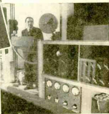
Below—A corner of the television control room, showing meters, etc., including film transmitter and its transmitter tube mounted in the oblong box at the left.
