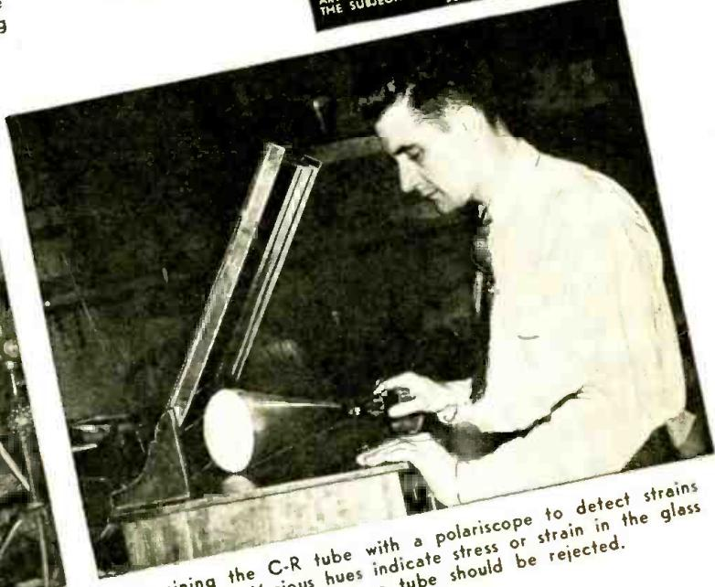
Examining the C-R tube with a polariscope to detect strains in the glass. Various hues indicate stress or strain in the glass and tell whether a tube should be rejected.
