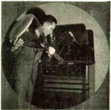
The set produces a black and white picture  $9'' \times 12''$  in size, and sells for about \$425.00. As can be seen in the picture, there are six controls for sight and sound —the latter coming through the grill below the control panel. While the set is designed for 405-line reception, it can be readjusted to operate on the 441-line pictures, which are the American standard.
