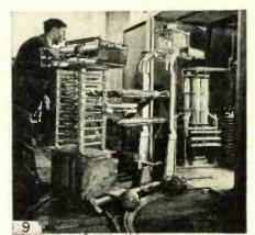
mitter normally works. The giant coils are for the final stage of the transmitter, smaller units, mounted on rubber-tired trucks, being used in the earlier stages.
