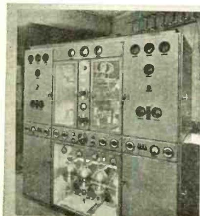
The 1 kW transmitter You have heard. The two crystal controlled oscillators corresponding to two wave-lengths are on both sides of the high level modulated power amplifier.
