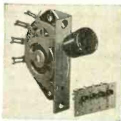
● A LOW capacity lever-action switch has just been announced by the Centralab concern. The switches are similar to toggle switches in their action, as far as the operating lever is concerned, but the contacts are more like those of the familiar rotary switches. They take up an
